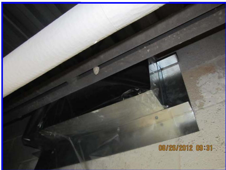
ROOM # 1-CONTAINMENT OF TRANSFER DUCT
